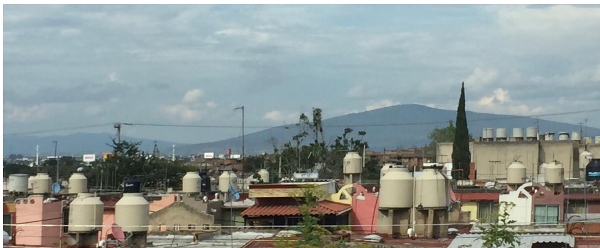
Figure 1. Typical rooftop tanks in Guadalajara
