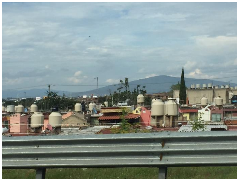
Figure 1. Typical rooftop tanks in Guadalajara
