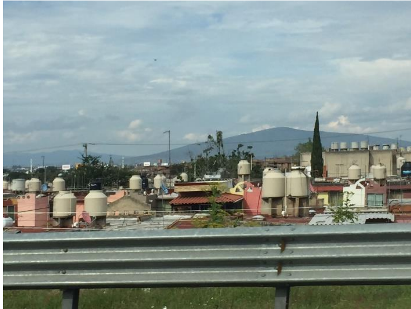
Figure 1. Typical rooftop tanks in Guadalajara
