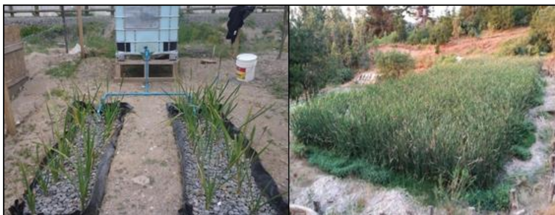
Figure 1. Wetlands of horizontal subsurface flow. (Left) Pilot wetlands, located in dependencies of the University of Bío Bío, Concepción. (Right) Real-scale wetland, located in the Recreational Center Ainahue, Hualqui.
