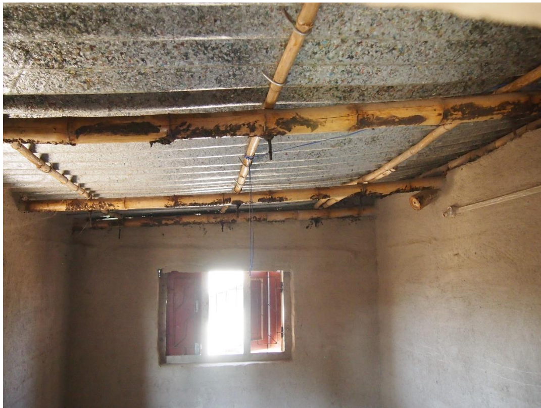
Figure 5: Interior of 'completed sustainable house' showing borer infested roof structure, imported Tetrapak roofing and windows without external overhang shading (as in adjoining school building)
