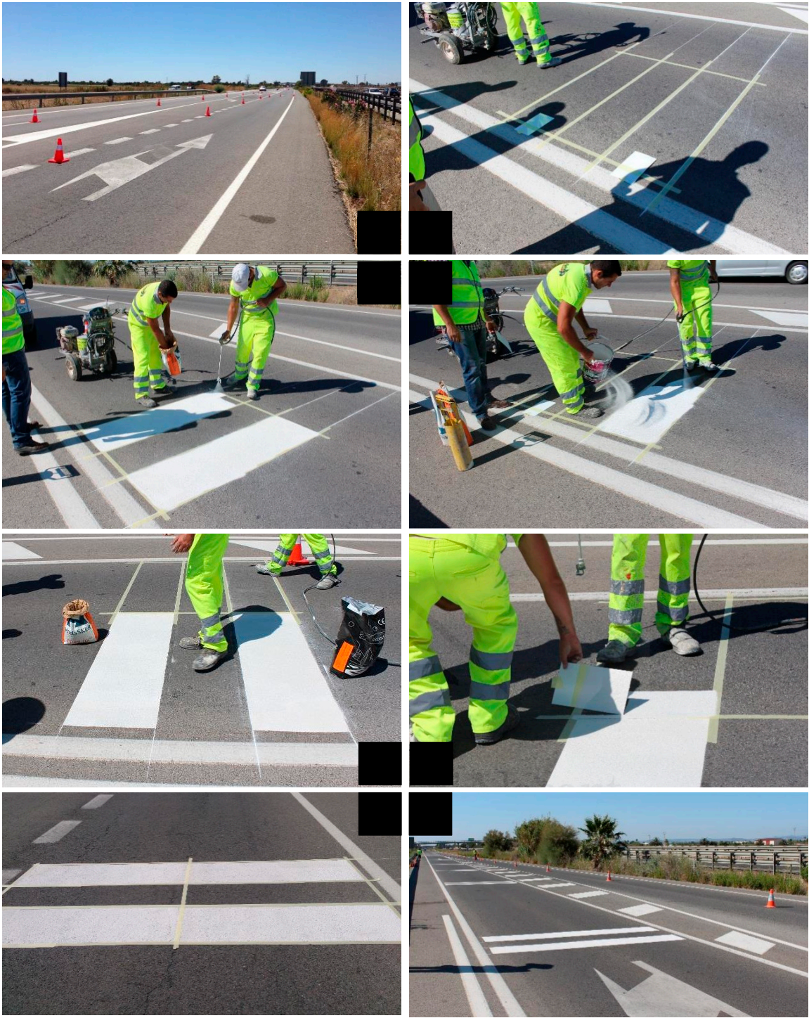
Figure 4. Sample fabrication process: (a) traffic diversion; (b) sample sketching with chalk and adhesive tape; (c) spraying of base material; (d) application of drop-on material; (e) in-situ test sample finished; (f) laboratory specimen fabrication; (g) transversal stripe completed; (h) finished test section, ready to be opened to traffic.
