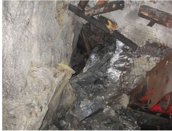
Fig. 3 The narrow coal pillar crushed by the mining stress
