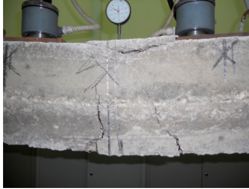
Figure 4. Dial displacement gauge position.
