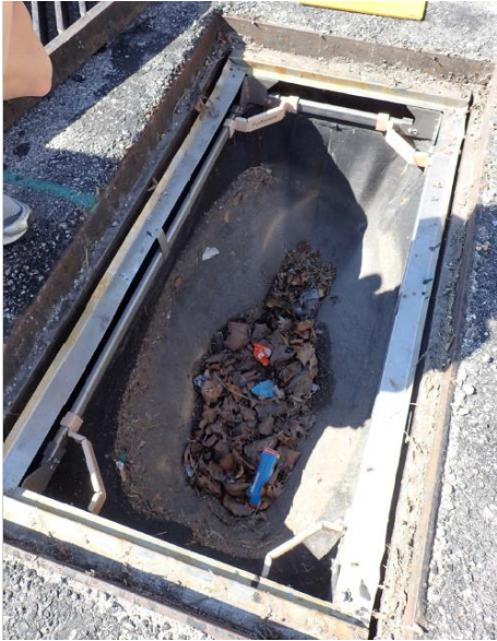
Figure 2. Trash guard installed in GI1 inlet structure (Date: October 18, 2016).
