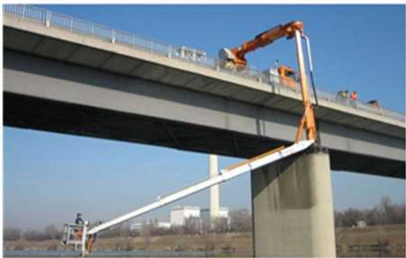
Figure 1. Close inspection using bridge inspection vehicle
