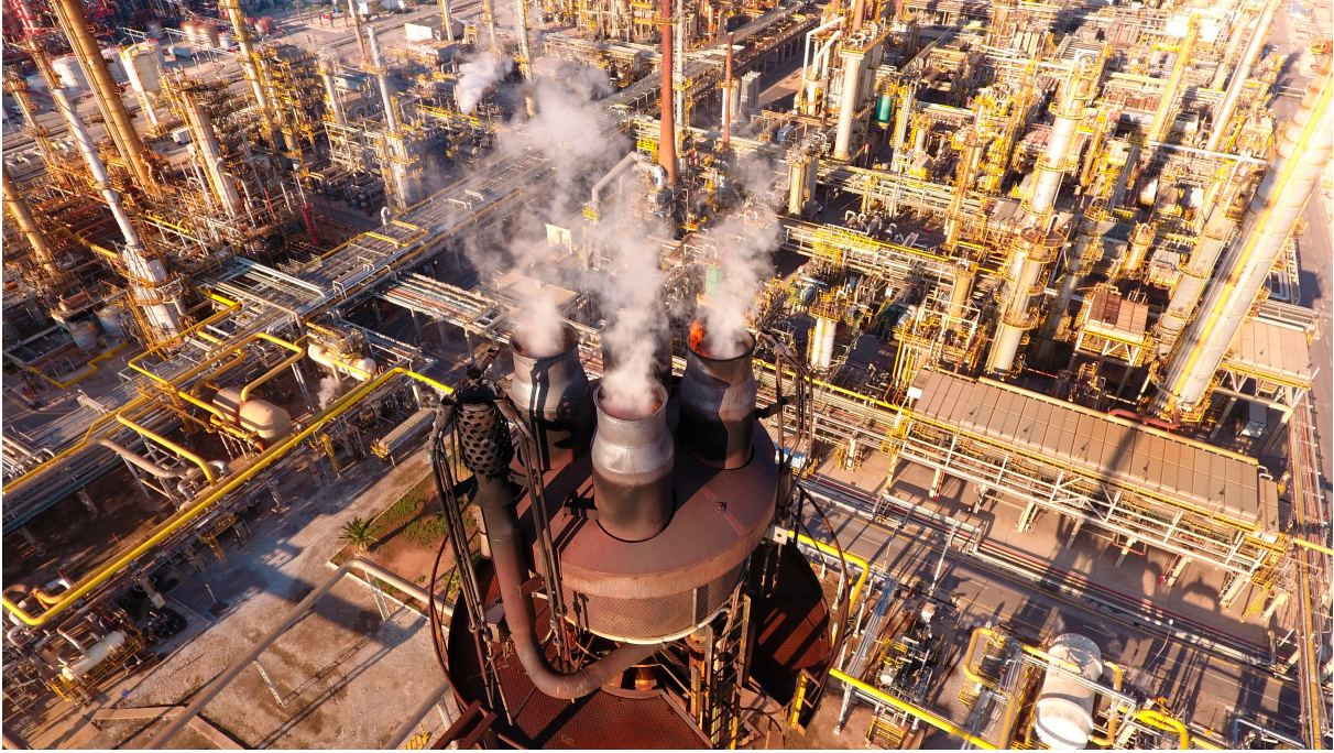
PHOTO 8.2 View from above of a burner in operation using drone inspection
