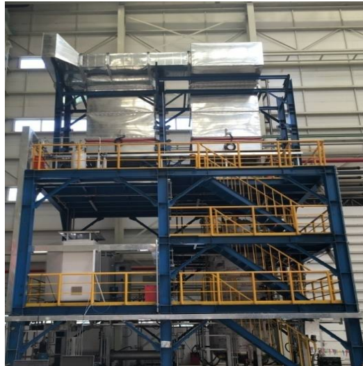
Figure 4. Overall view of experiment facility
