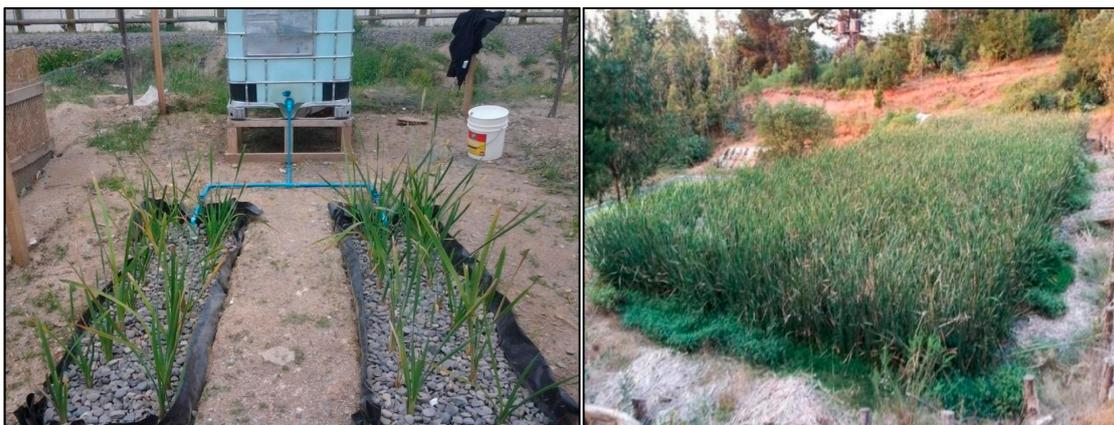
Figure N°1. Wetlands of horizontal subsurface flow.
