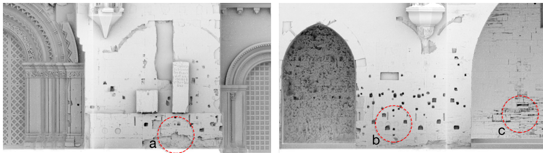
Figure 4. 2D raster from an environmental occlusion generated in 3D: (a) loss of material, (b) holes and alterations of the stone, and (c) disintegration of stone.
