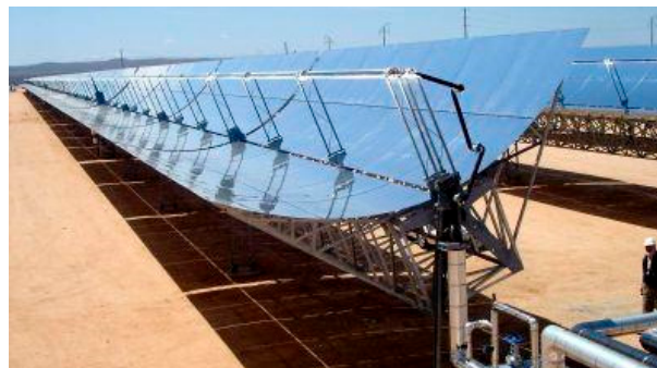
Figure 7. Parabolic trough collector. Source: Enerstar.
