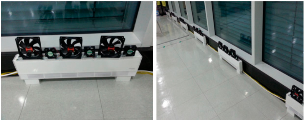
Figure 10 Installation View of Equipment System with Added Convector + Circulating Fan
