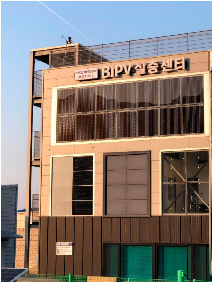
Figure 1. Full-scale mock-up building with various multifunctional prefabricated façade cladding.
