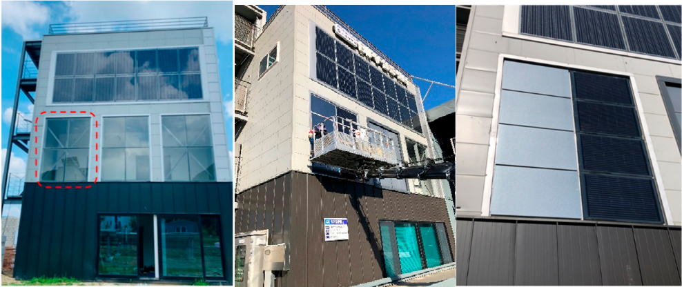
Figure 3. Full-scale mock-up building (left) and BIPV module installation (middle) and completed BIPV system (right).
