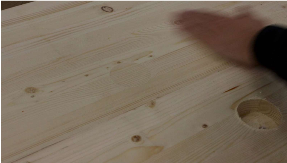
Figure 17. Close-up of the restored surface of the wooden glulam beam.
