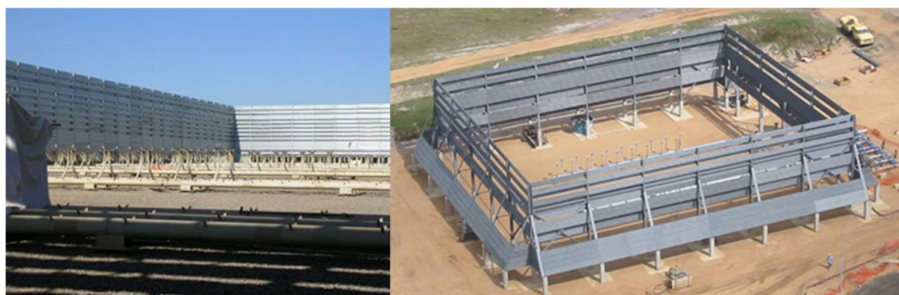
Figure 6. Effective wind fence designs protect surrounding equipment and personnel from high radiation flux while providing necessary air for efficient combustion (courtesy Zeeco, Inc.) [2].
