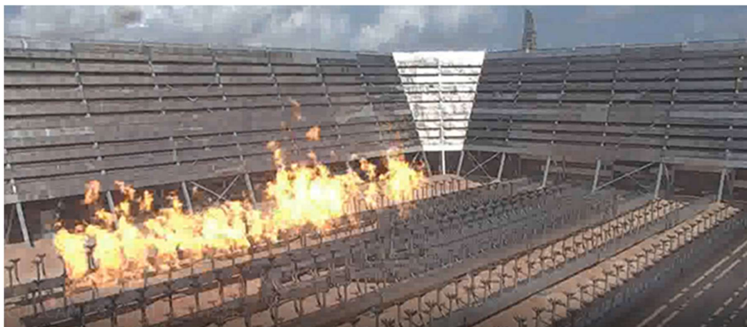
Figure 7. MPGF located in Port Arthur Texas, USA, stages 1 and 2 burning (courtesy Zeeco, Inc.) [5].
