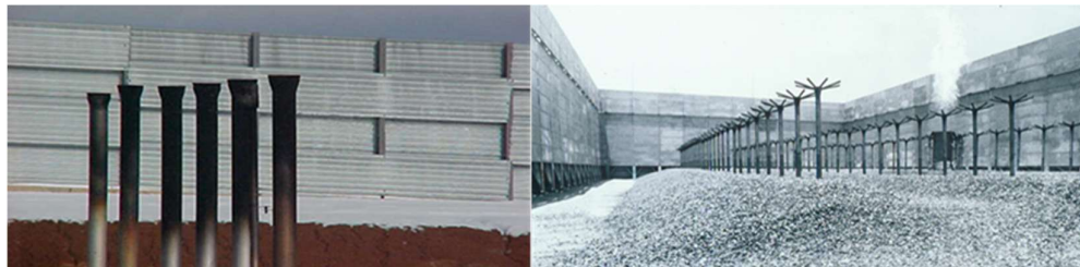
Figure 1. Early Multi-Point Ground Flare designs circa 1950-2000 (courtesy Zeeco, Inc.).
