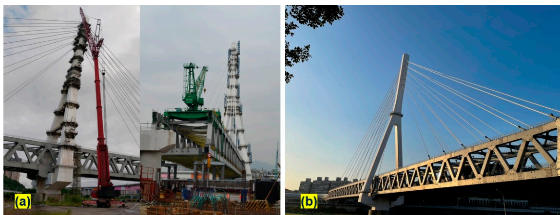
Figure 10. The Anhsin Bridge (a) during construction and (b) after completion.
