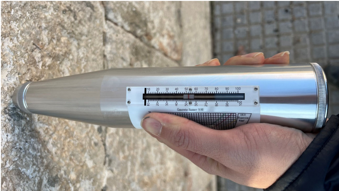
Figure 6. Measurement of the compressive strength of the Cathedral Tower’s limestone using a Schmidt hammer, taken from the first ashlars on the west façade (photograph by the author).
