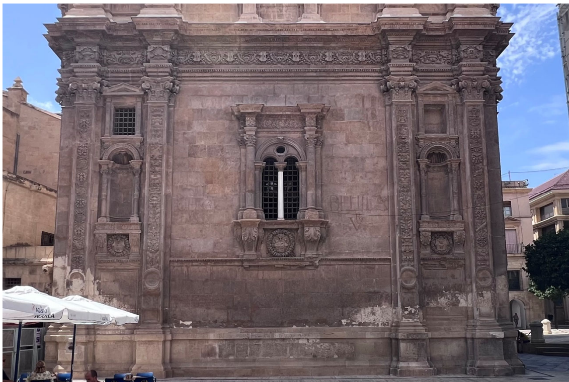
Figure 3. First tier of the bell tower of Murcia Cathedral, east façade (photograph by the author).
