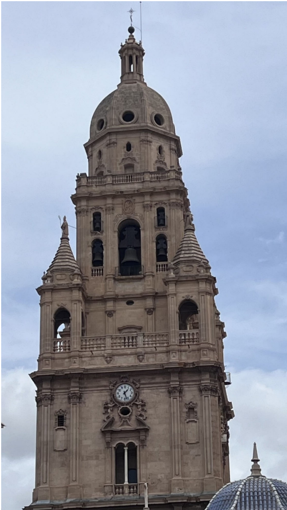
Figure 5. Third tier, conjuratorios, and bell chamber of the Cathedral Tower, west façade (photograph by the author).
