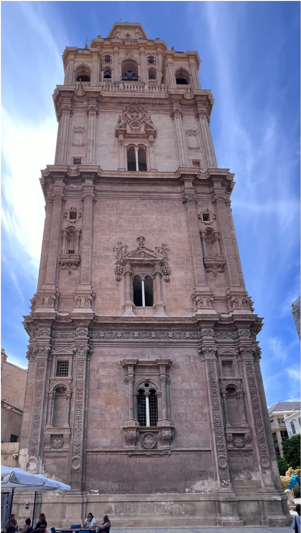
Figure 9. Eastern elevation of the tower, showing the same deviations and corrective alignments introduced as construction advanced (photograph by the author).
