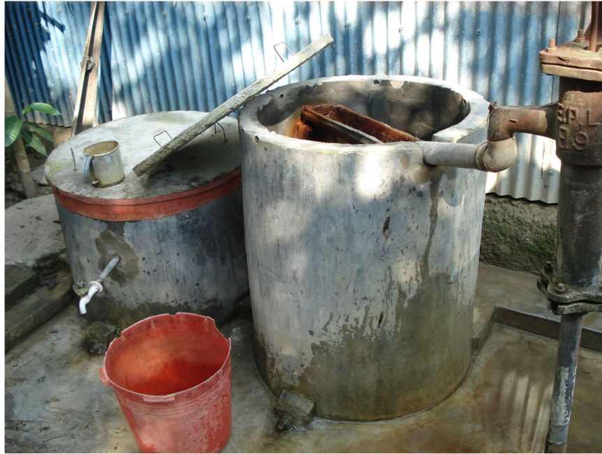
Figure 3. Photo of an Arsenic Iron Removal Plant in Bangladesh (Brennan & McBean, 2010a).
