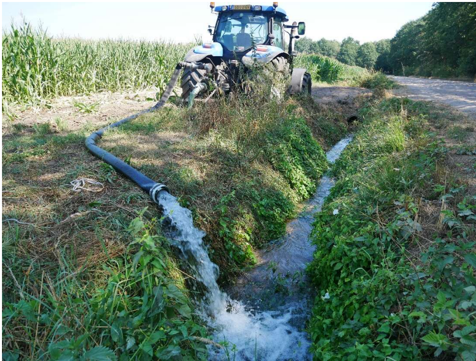
Figure A4. Groundwater influx to the Reusel by pumping in a ditch upstream of Wellenseind, pumping continued until september (23th of July, picture: M. Schiphouwer).
