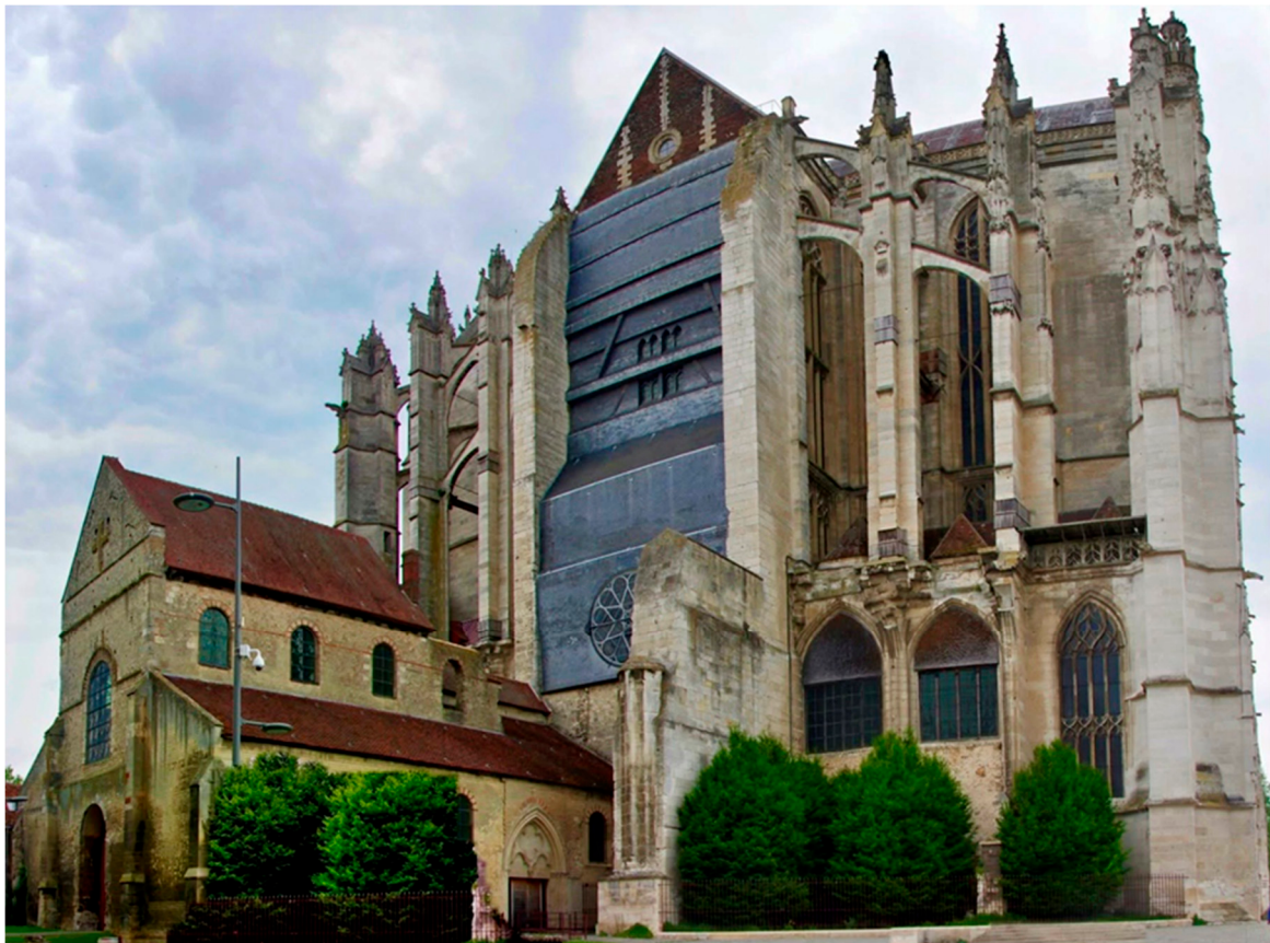
Figure 2. Overall view of the southern façade of Beauvais Cathedral, highlighting the missing nave, the incomplete transept, and the adjacent preexisting structure, the Basse-Œuvre (photograph by the author).
