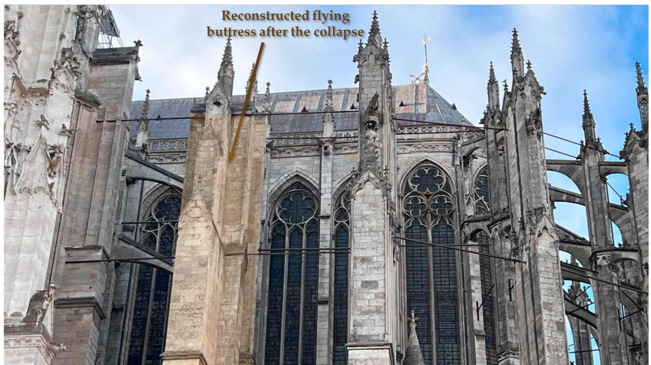
Figure 7. General view of the exterior of Beauvais Cathedral's choir, showing the reconstructed and heightened flying buttress following the 1284 collapse (graph by the author).
