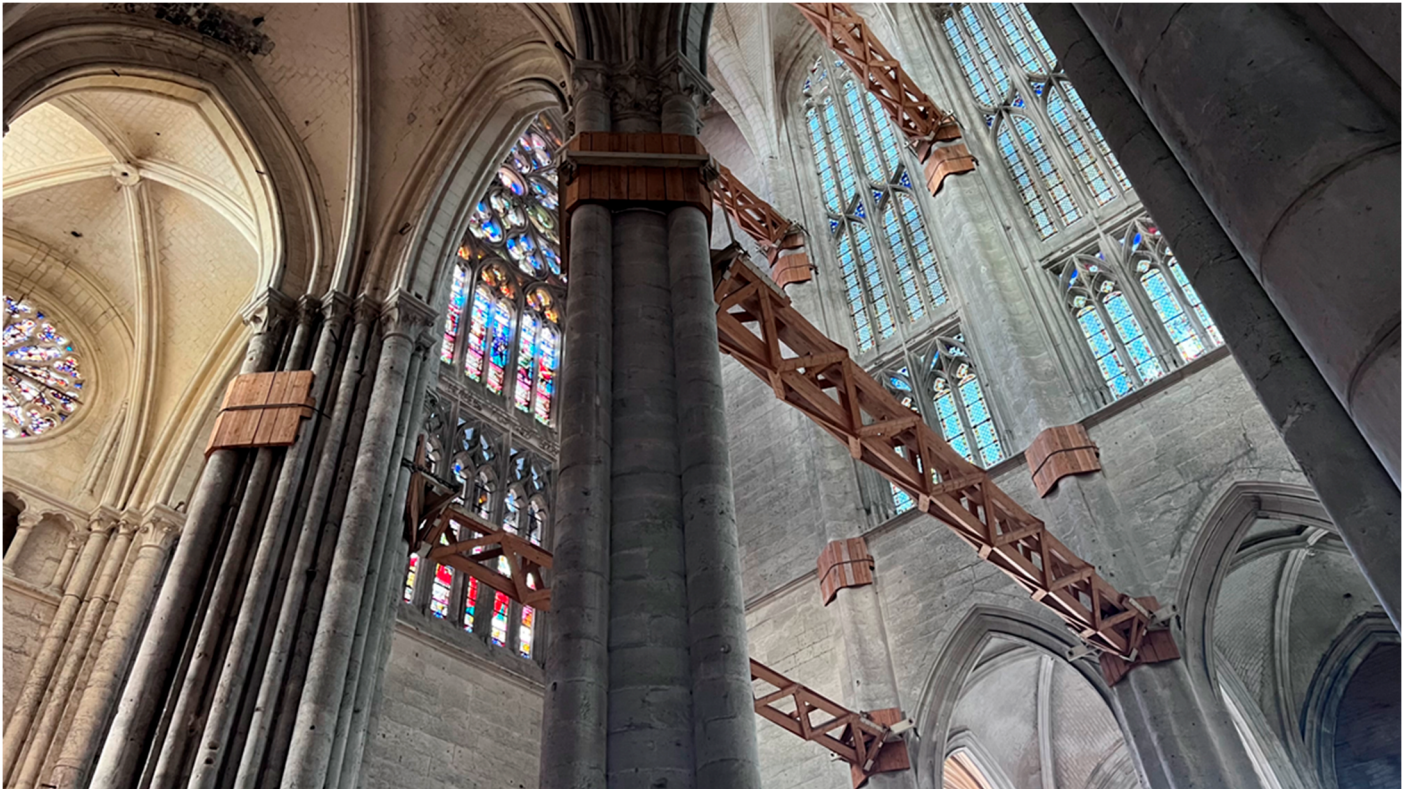
Figure 12. Interior view of Beauvais Cathedral, showing the wooden tie beams installed for structural support (photograph by the author).
