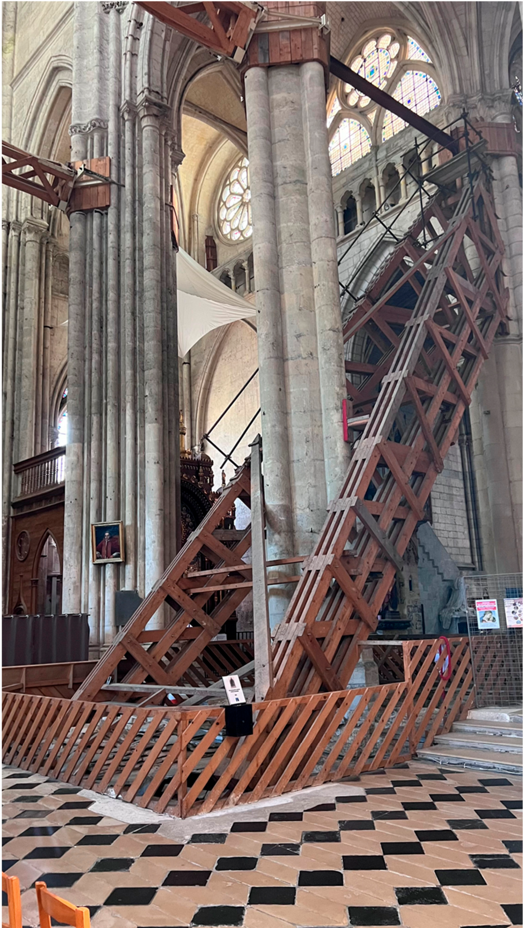
Figure 13. Wooden stabilization system installed inside Beauvais Cathedral, at the junction of the north transept and the choir nave (photograph by the author).
