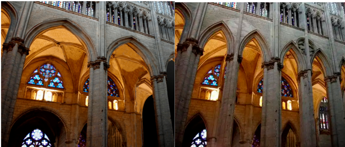
Figure 11. Comparison between the pre-collapse state (reconstruction, left) and the post-collapse state (right) of the Beauvais Cathedral choir after the 1284 collapse, highlighting the reinforcement achieved through the duplication of piers (diagrams by l'Association Beauvais Cathédrale [15]).
