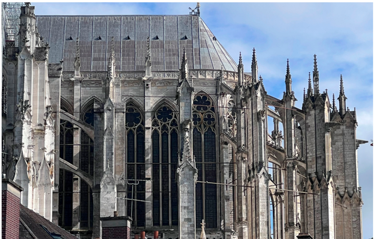
Figure 6. General view of the exterior of Beauvais Cathedral's choir, showing the area where the collapse occurred (photograph by the author).
