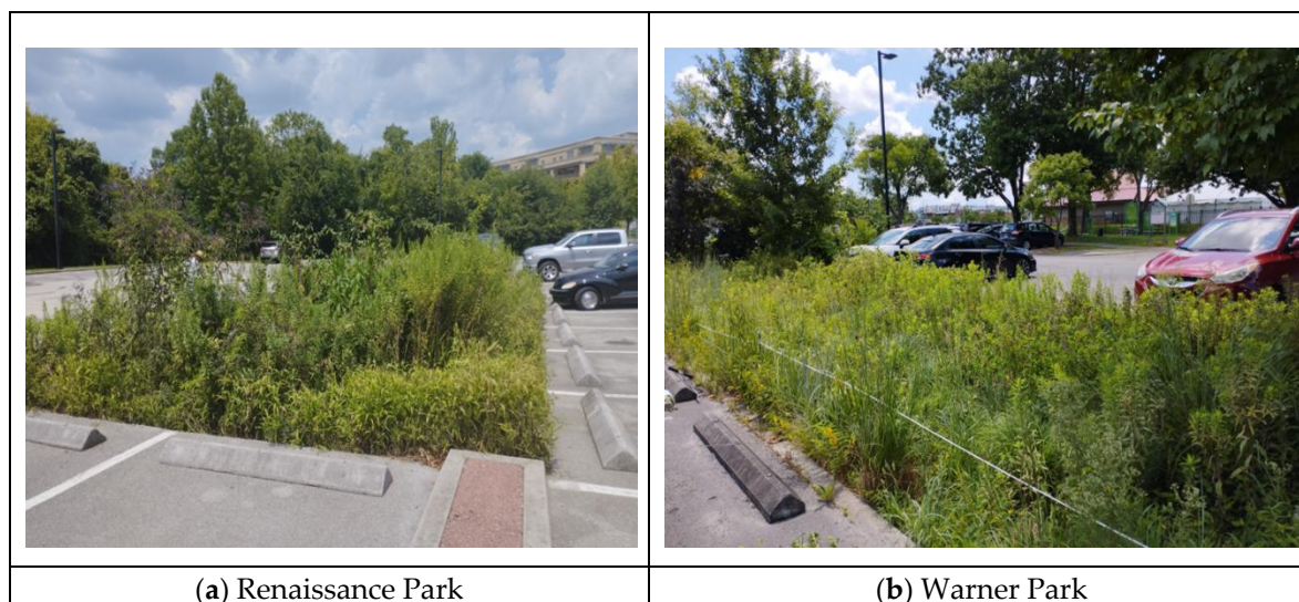
Figure 1. Bioretention media with native plants (a) Renaissance Park (b) Warner Park.
