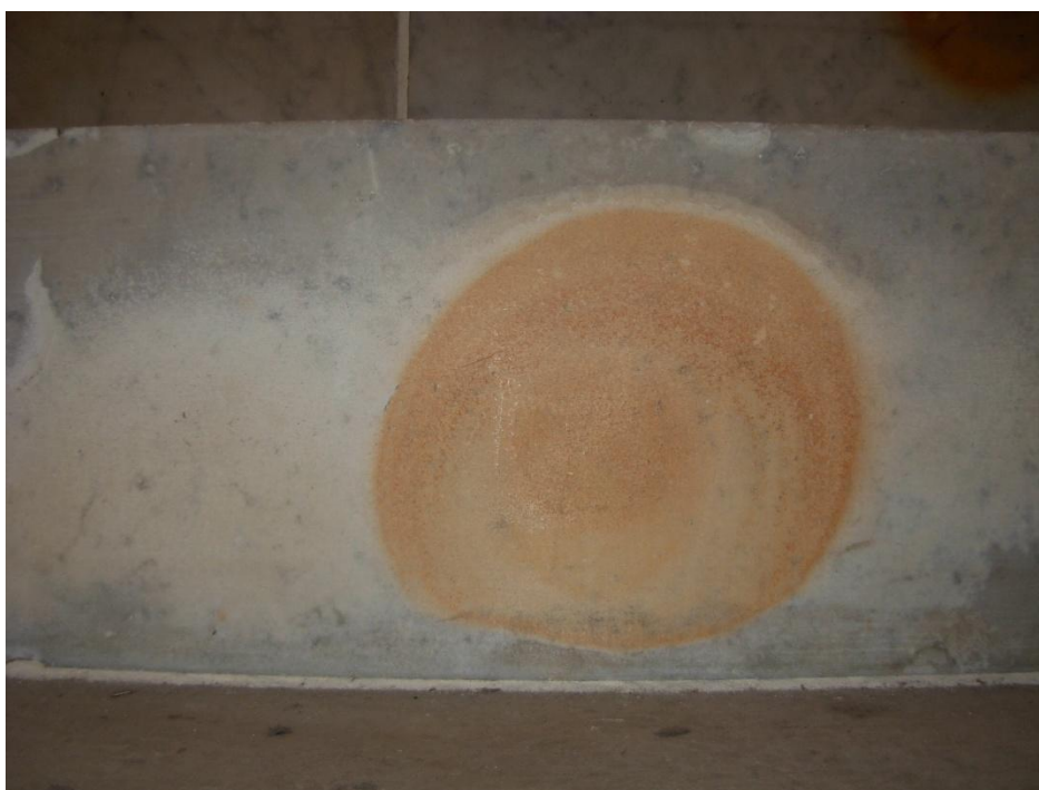
Figure 12. Red spots formation due to colloidal iron oxide radial diffusion.
