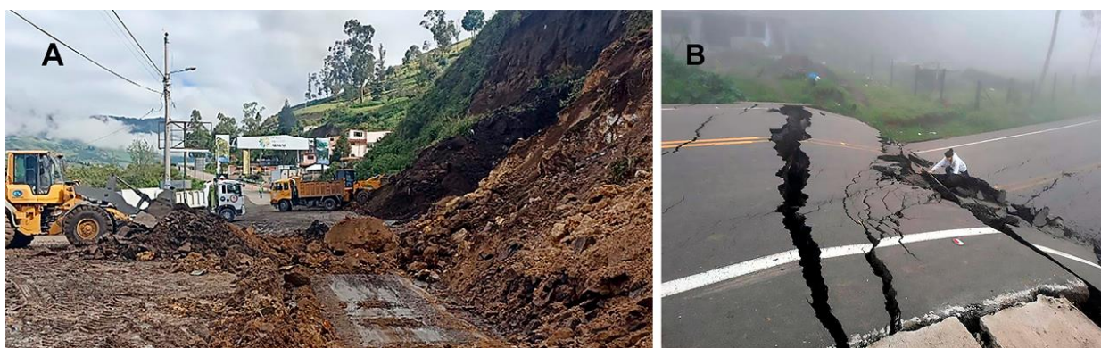
Figure 9. (A) Government machinery works to clean and open the E-35 Road, south of the Don Fausto restaurant, in the casual sector, February 19, 2023 [30]. (B) Impressive open cracks and vertical displacement (over four meters) 50 m North of the Don Fausto restaurant. The picture was granted by S. Berrones, a geologist, who took it on 26th Mars 2023 in the morning, a few hours before the event happened.
