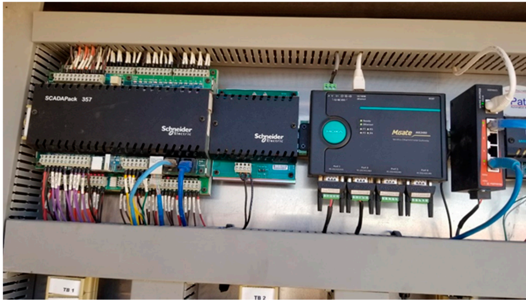
Figure 6. SCADA Hardware-BPX Tank Battery Site in Orla, TX.
