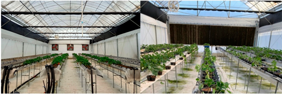
Figure 1. The evaporative greenhouse equipped with a pad-and-fan system. The exhaust blowers draw in outdoor air through water-cooling pad to lower the room’s temperature.
