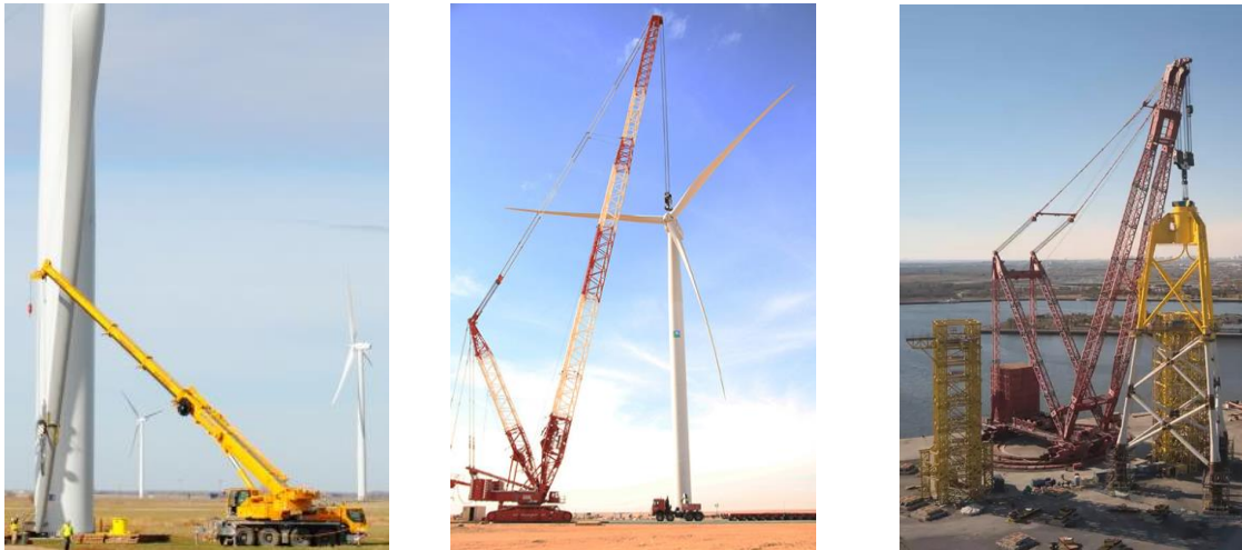
Small Medium Large Truck-type for small components lifts and as an auxiliary during large lifts. Crawler-type for small and medium components lifts Ring-type for large lifts and at great heights
