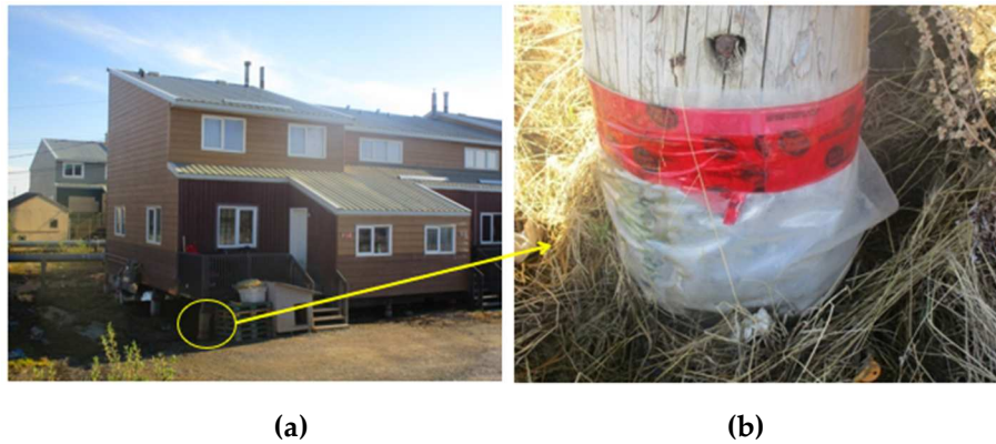
Figure 10. (a) residential construction using a timber pile foundation in Inuvik, NWT, Canada; (b) tuck tape protecting timber from the water.
