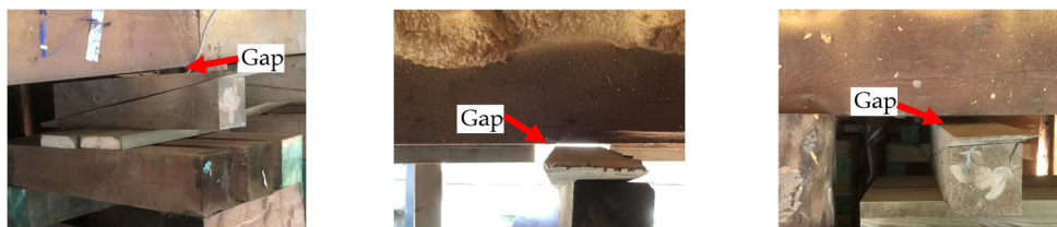
Figure 6. Vertical gaps caused by the seasonal weather between the wood block wedge and building base floor beam.
