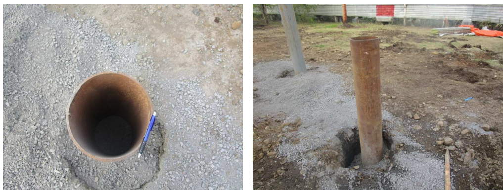
Figure 11. Typical steel pipe pile foundation in Permafrost with backfill.
