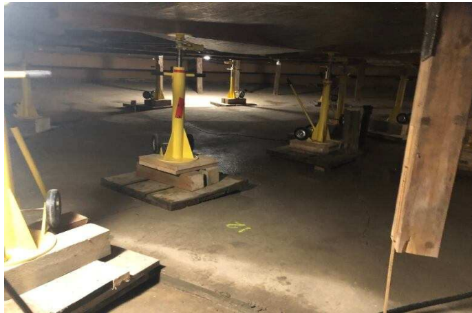
Figure 7. The use of screw jacks in permafrost can be seen in the construction of the "igloo" church in Inuvik, Canada [20].
