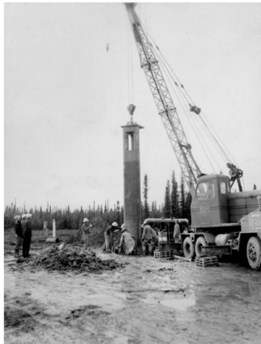
Figure 12. Installation of the first thermopile in 1960 [27].
