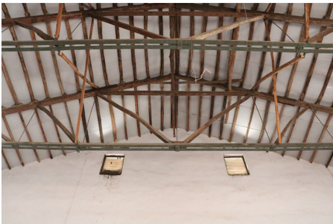
Figure 10. Truss structure of Weixing Commune hall
