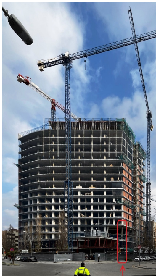
Figure 2. Image of the construction process of the hotel already finished in January 2022. Indicated with a red rectangle the vertical provisional column that has not yet been removed, can be seen.
