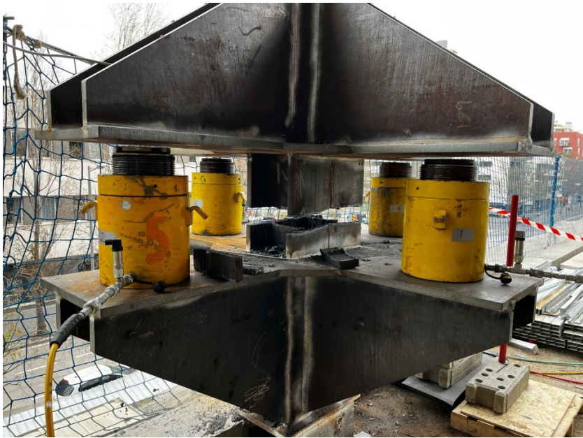
Figure 6. Image of the system after the column is cut and separated from the system. In the top head of each piston a space is visible. The transducers were removed before this photo was made.
