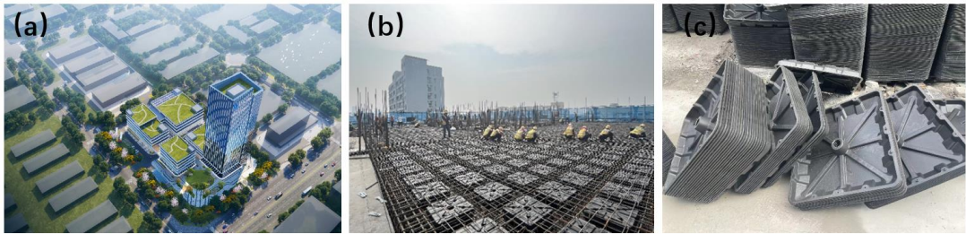
Figure 1. Schematic Diagram of the Box-shaped Core Mold and Its Layout in the Hollow Floor Slab. (a) Architectural rendering; (b) Floor slab layout; (c) Core Mold Schematic Diagram.
