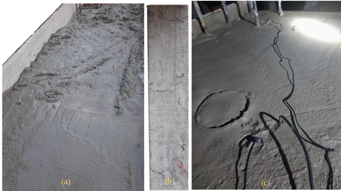
Figure 7. (a) slab surface preparation, (b) structural column, (c) slab with sensor installed.
