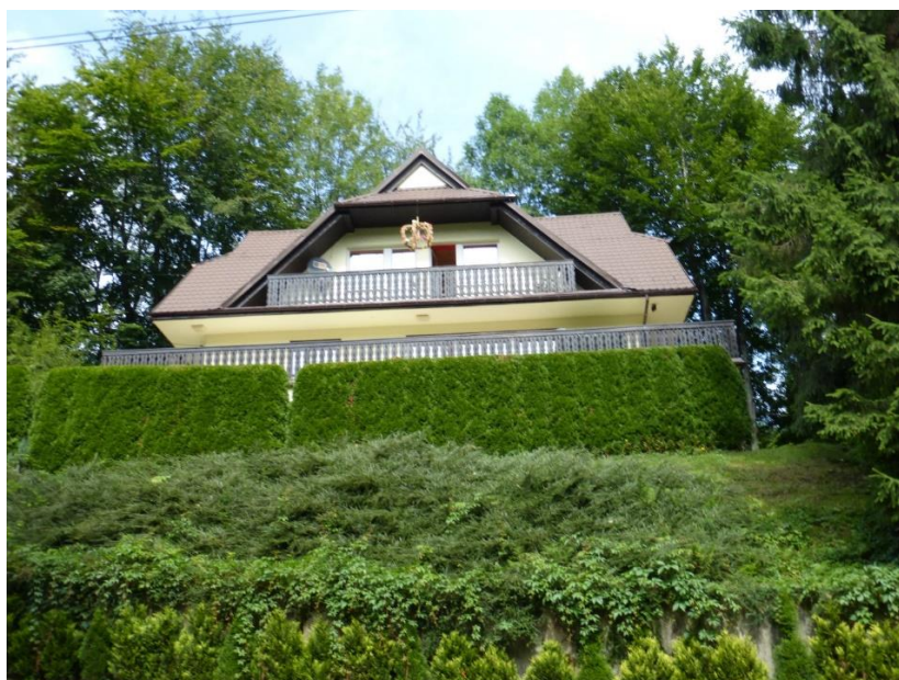
Figure 4. A heavy masonry recreational house, founded on a steep mountain slope in Brenna. At the bottom of the photo, there are large retaining walls overgrown with vegetation. Source: author's archive.
