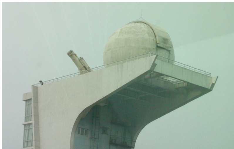
Figure 8. The tower of Huairou with the sliding dome, the MCS Telescope and the SC 11" telescope to the left, during the Venus' transit. The sky remained hazy all day.
