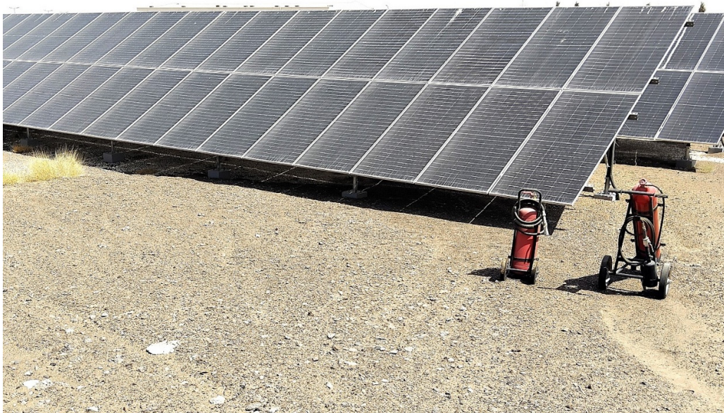
Figure 1. Photo of a bifacial photovoltaic system with a soil ground with a dark color, thus allowing very low albedo (photo taken by the author).
