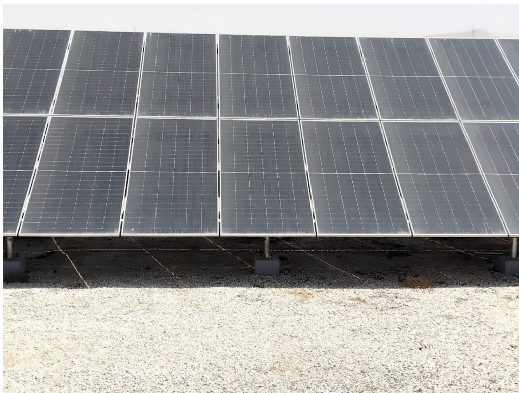
Figure 2. Photo of a bifacial photovoltaic system with the ground covered intentionally by gravel to improve light reflection, thus allowing high albedo (photo taken by the author).
