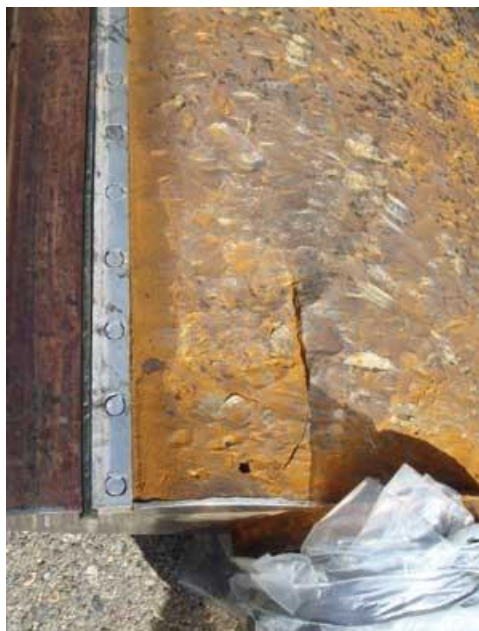
Figure 4. The skin plate damages of a guided vane of G.M. Shrum, BC Hydro [7].
