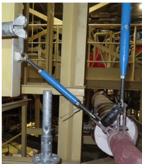
Figure 1. typical sway struts (blue).
