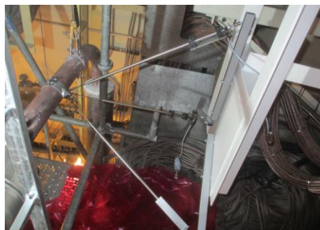
Figure 9. Mounting of the inductive displacement transducers on the pipe at the observation point Q.
