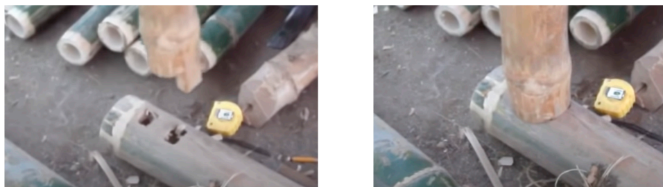
Figure 12. Mortise-tenon joints [72].
