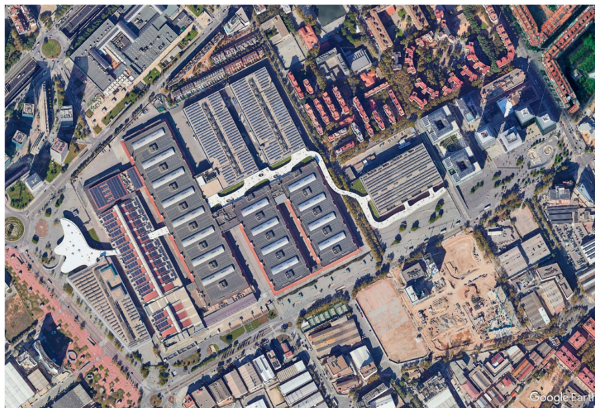
Figure 1. Aerial view of the Fira de la Gran Vía in Barcelona. The three buildings whose roofs display a sequence of rectangle–square–rectangle forms are, from left to right, Halls 3 (4 ha), 4 (3.4 ha), and 6 (3.5 ha). Image: Google Earth.
