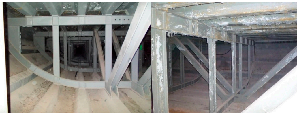
Figure 4. Interior of the steel superstructure showing longitudinal and transverse stiffening trusses, with shell sheets reinforced by longitudinal trapezoidal ribs.
