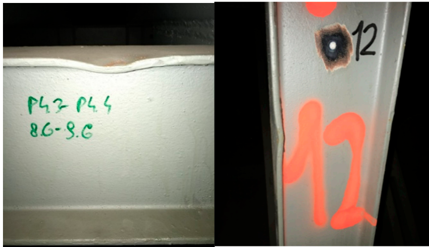
Figure 5. Local plastic deformations of the upper chord (left) and post (right) of the cross-beams.
