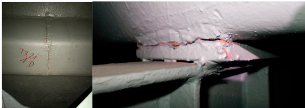
Figure 6. Typical weld cracks in the butt joints of longitudinal ribs (left) and an example of a crack in the fillet weld connecting the longitudinal rib to the upper chord of the cross-beam (right).
