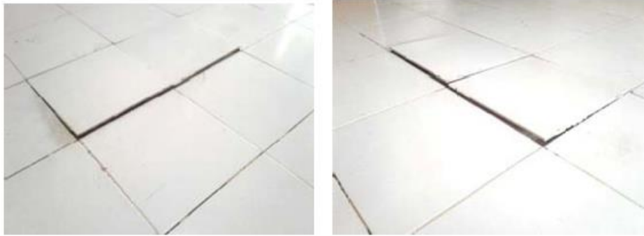
Figure 8. Ceramic Fractured on Floor.
