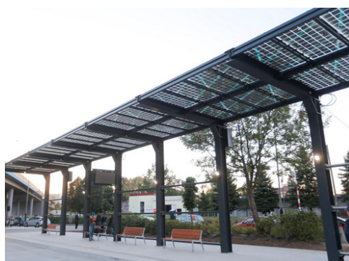
Figure 1. The object of the study – the platform of the Local Railway Station in Rzeszów (Poland).
