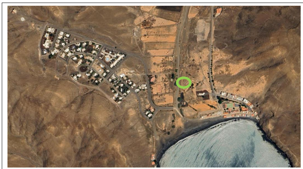
Figure 1. Situation of depuration plant within the centre of village (Green Circle). Note the arid conditions, the vicinity of sea and the reduced size of the settlement.
