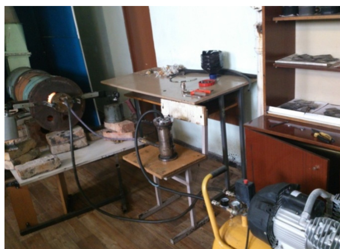
Figure 8. External view of the coal-water combustion plant.
