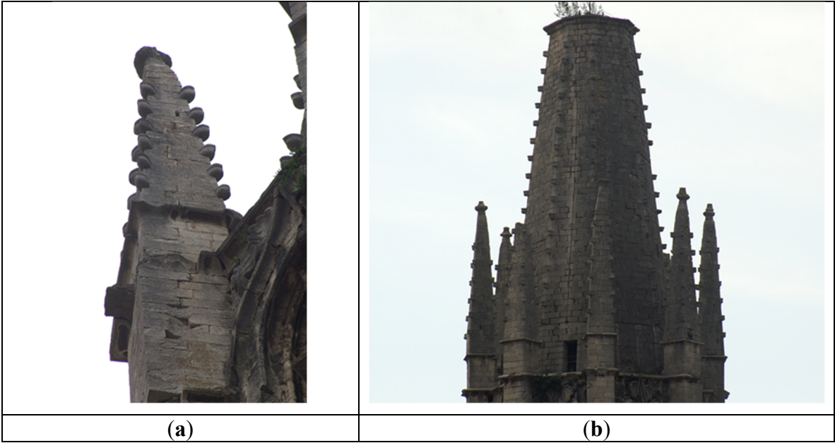
Figure 2. Truncated spire and pinnacles of Saint Félix church: (a) Detail of vertical deformation of pinnacle; (b) General view of deformation of pinnacles.
