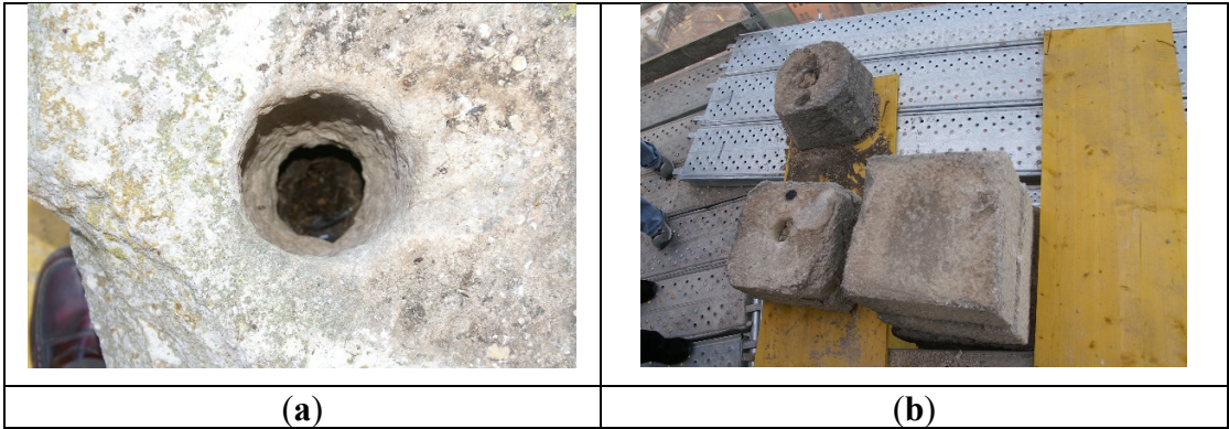
Figure 1. View of the hole where the wooden log was formerly allocated: (a) Whole at the top piece of pinnacle (b) Pieces of the pinnacle disassembled.
