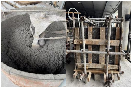
Figure 6. The sample of mass concrete during construction.
