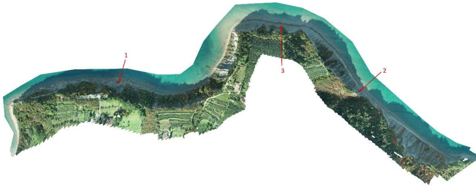
Figure 12. Selected areas of rockfalls.
