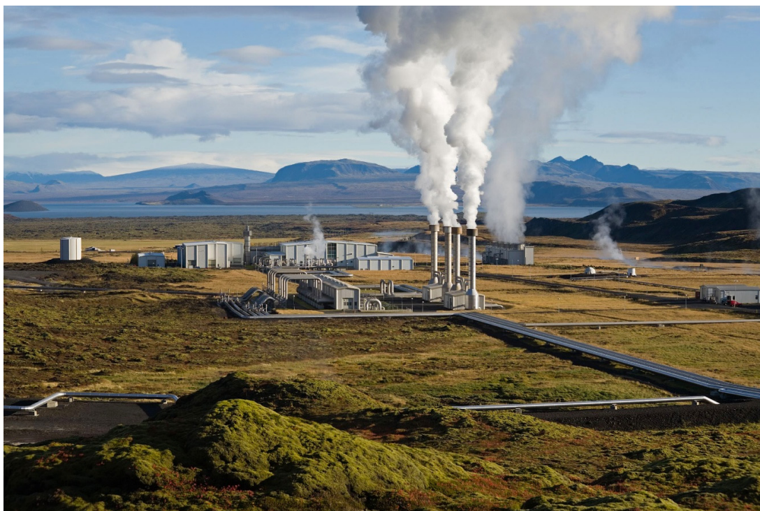
Figure 6. The Nesjavellir power plant near Þingvellir ( https://de.wikipedia.org/wiki/Nesjavellir-Kraftwerk ) is the largest geothermal power plant in Iceland. It provides 120 MW of electrical energy and 300 MW of thermal energy but has been able to do so for only approximately 30 years since 1990, after which its output has steadily decreased. With this electrical output, only as much CO 2 would theoretically be possible to extract from the air and become stored in the ground as a small 20 MW conventional power plant generates CO 2 .
